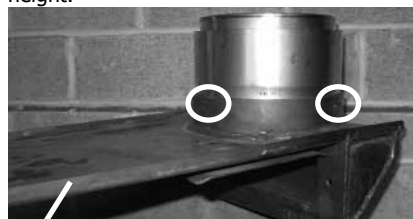
Diagram 2 Flue Adaptor
